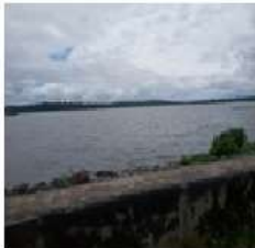
PLATE 5: DOWN STREAM OF ERO WATER DAM
