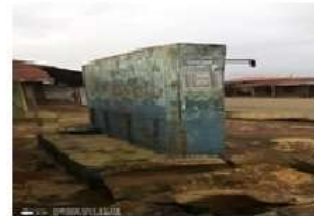
PLATE 7: MORIBOUND MDGs WATER PROJECT AT ADO-EKITI
