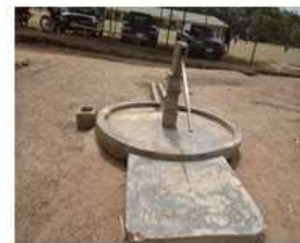
PLATE 10: ABADONED HAND PUMP WELL WATER AT ADO- EKITI
