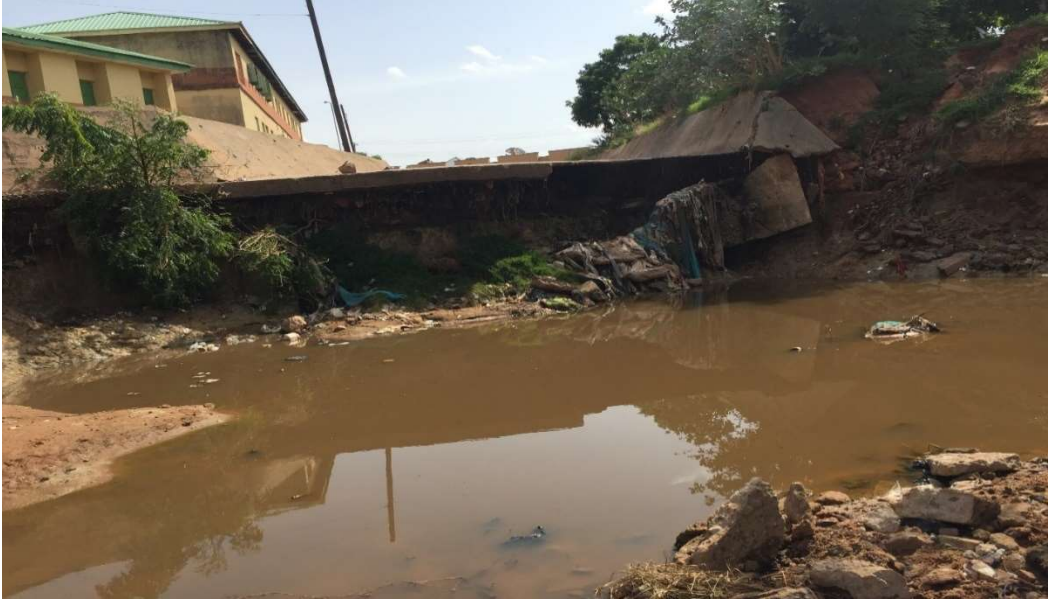
Plate 3: Improperly terminated drain system at the head of the extensive gully behind the Gombe State University
